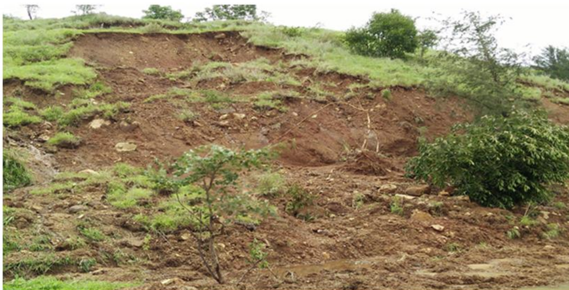
Fig. 5 Jotiba-Kerli road section slumping movement of weathered lava flow
