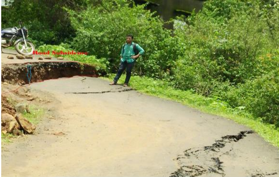
Fig. 6 Slumping movement occurs near Somwarpeth Panhala hill.
